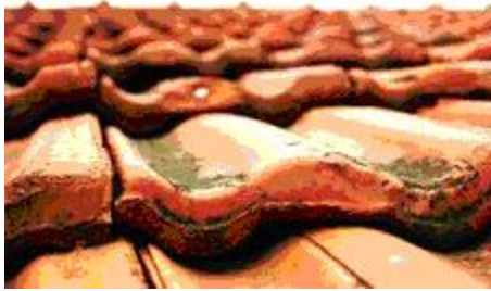
Asbestos cement roofing shingles
